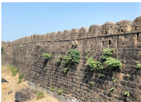
Fig.no.5 Fortified wall with merlon (Source- Author)
