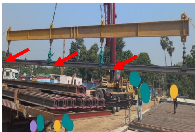
Figure 2 – Four Cam locks used while rail unloading
