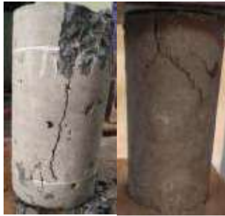
Fig.4 Failure Pattern of Cylinder Specimens
