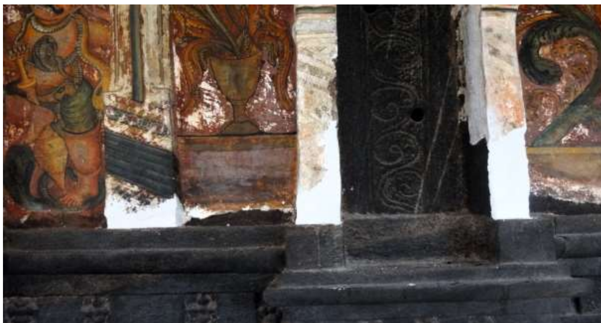
Trial and error experimentation on micro level phase (a) Lime and Cissus glauca roxb extract (b) Lime with Bael fruit extract (c) Lime mixed-up with tender coconut water applied on the walls
