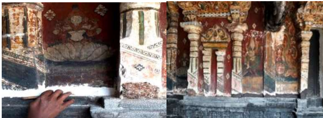
(a) Filling work on the cracked base of the murals at Erattayappan at macro level execution phase (b) Further lime coating on the cracked fissures and grooves to accomplish white lime texture for feasible colour reintegration works
