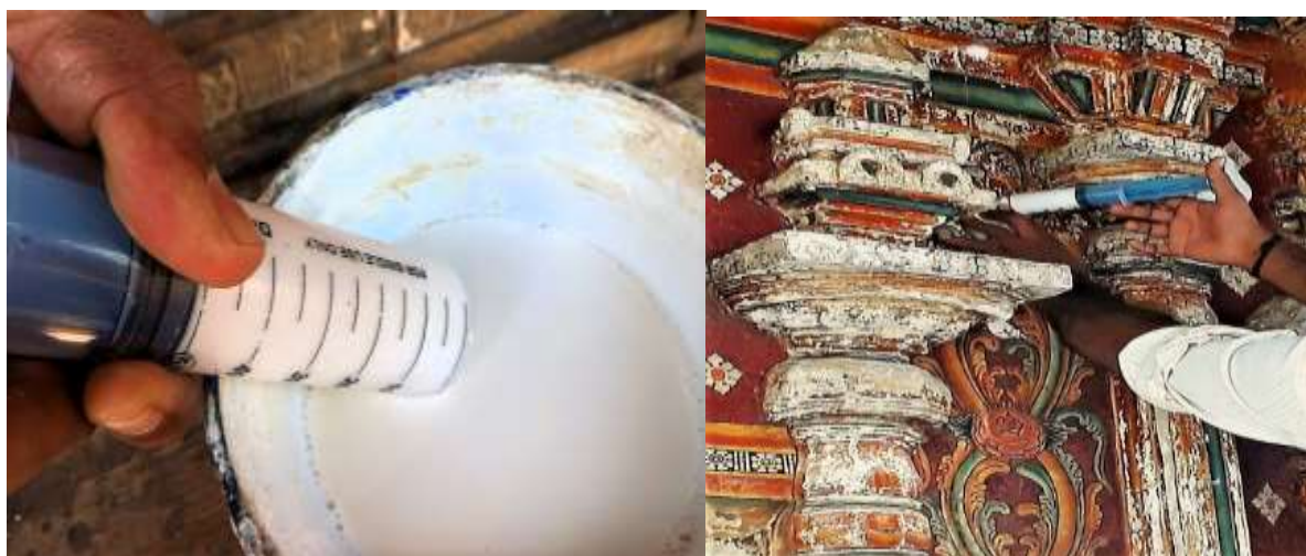
(a) Filling work on the minor cracks and fissures of the murals at Erattayappan at by injection method- Diluted lime with binder extract taken in syringe for injection into the micro fissures under consideration (b) Injection of lime into the micro fissures to fill the hollow area of the ground
